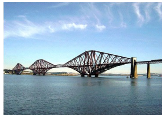
Bracket Bridge, Railway Bridge, Forth.
